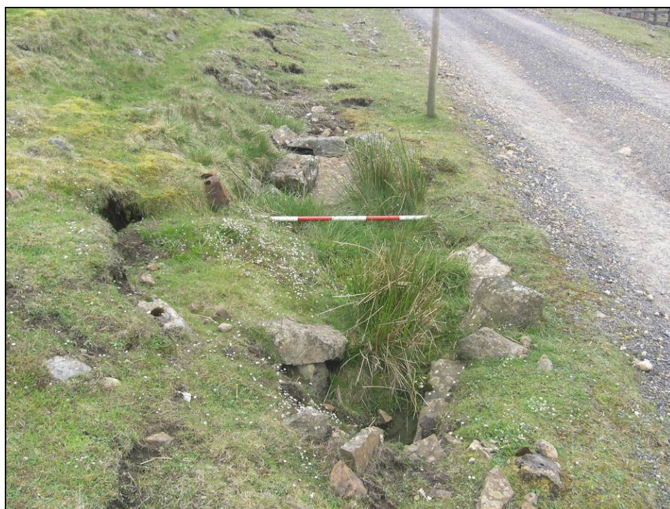
Plate 30: Collapse of leat (2460) adjacent to valve housing.
