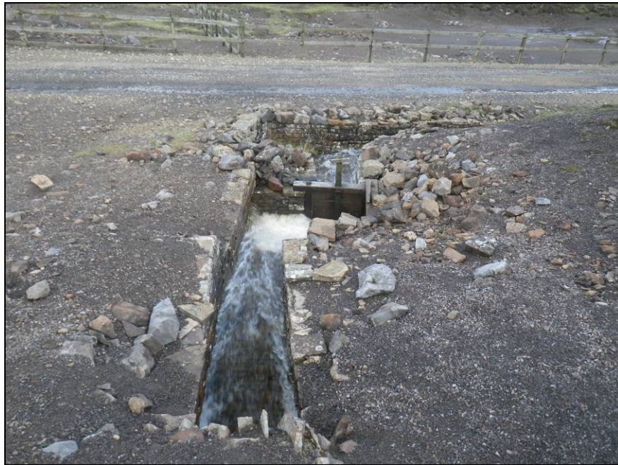
Plate 51: Water flowing from culvert ( 2462 ) to series of sluice gates and changing course to the northwest.
