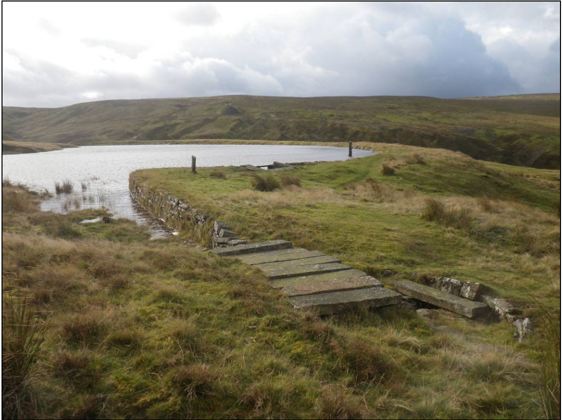
Plate 8: Overflow (0032) to the right of the image with the continuation of leat (0029) into the reservoir.
