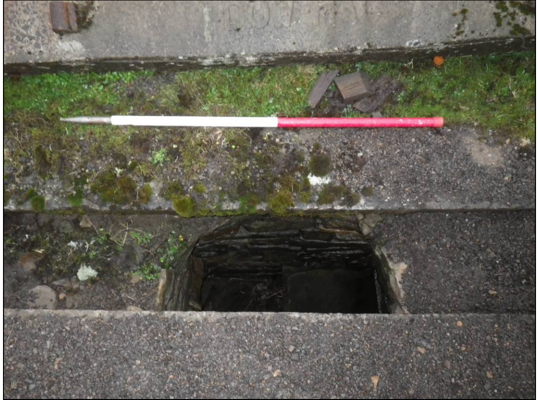
Plate 63: Railway sleeper removed at (2445) to reveal inspection hatch for (2575).
