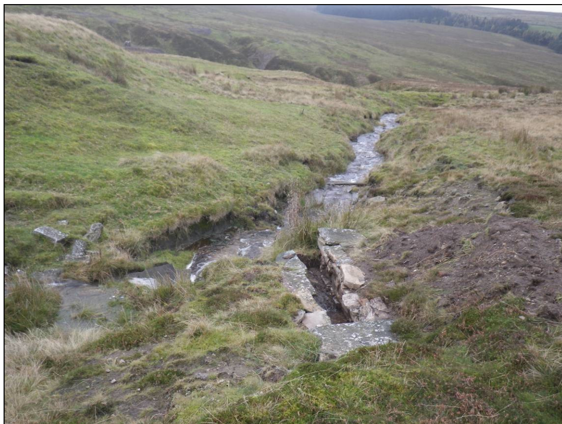
Plate 17: Culvert (2440) facing southwest showing collapsed retaining walls.
