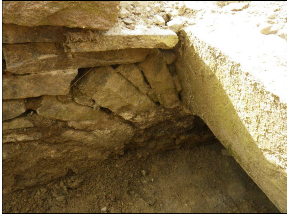
Plate 35: Trench 13, facing south showing section of blocked arching.
