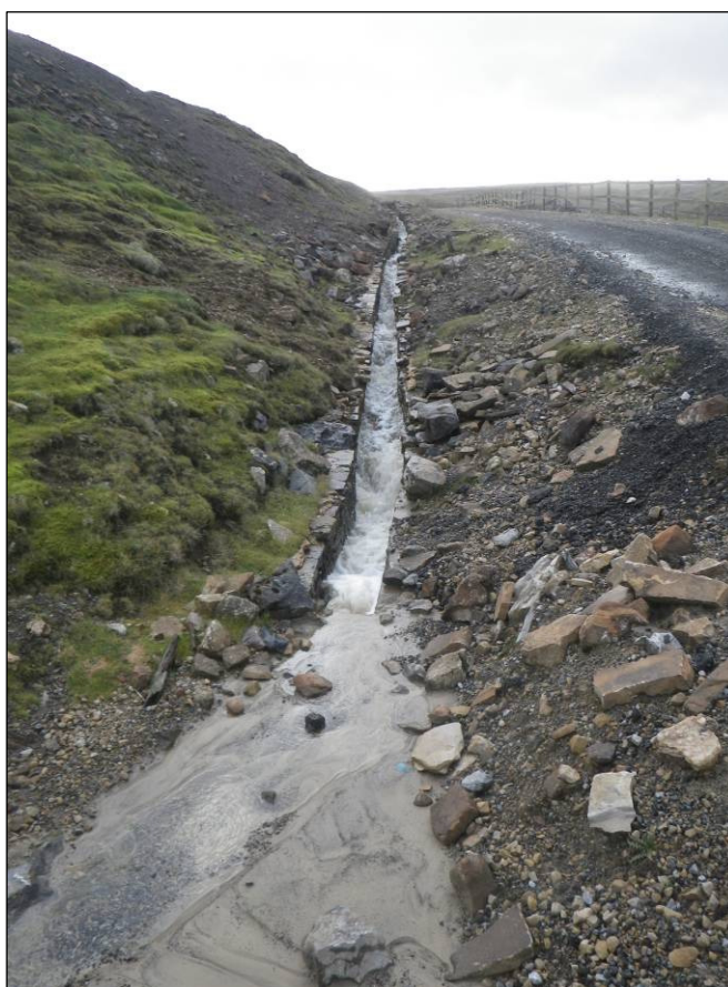
Plate 53: Water diverted into leat (2462) from sluice gates. Note water pooling on surface and flowing into leat at bottom of image.
