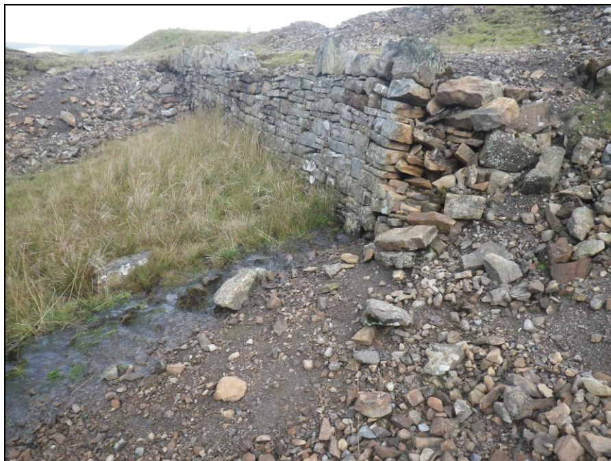
Plate 31: Water poaching through base of retaining wall and heading down slope to the southwest.
