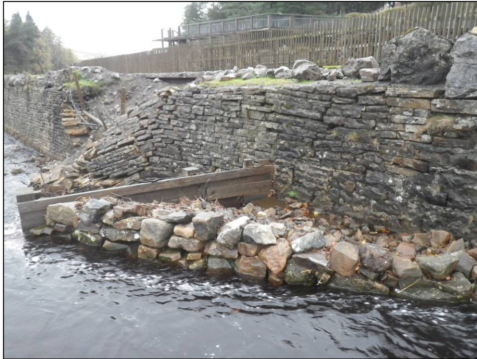
Plate 62: Main flow of water diverted away from collapsed section of retaining wall.
