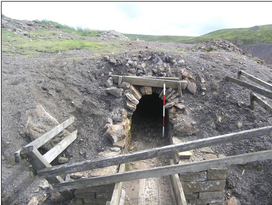
Plate 28: Culvert (2573) as it crosses launder (2574) to meet culvert (2575).
