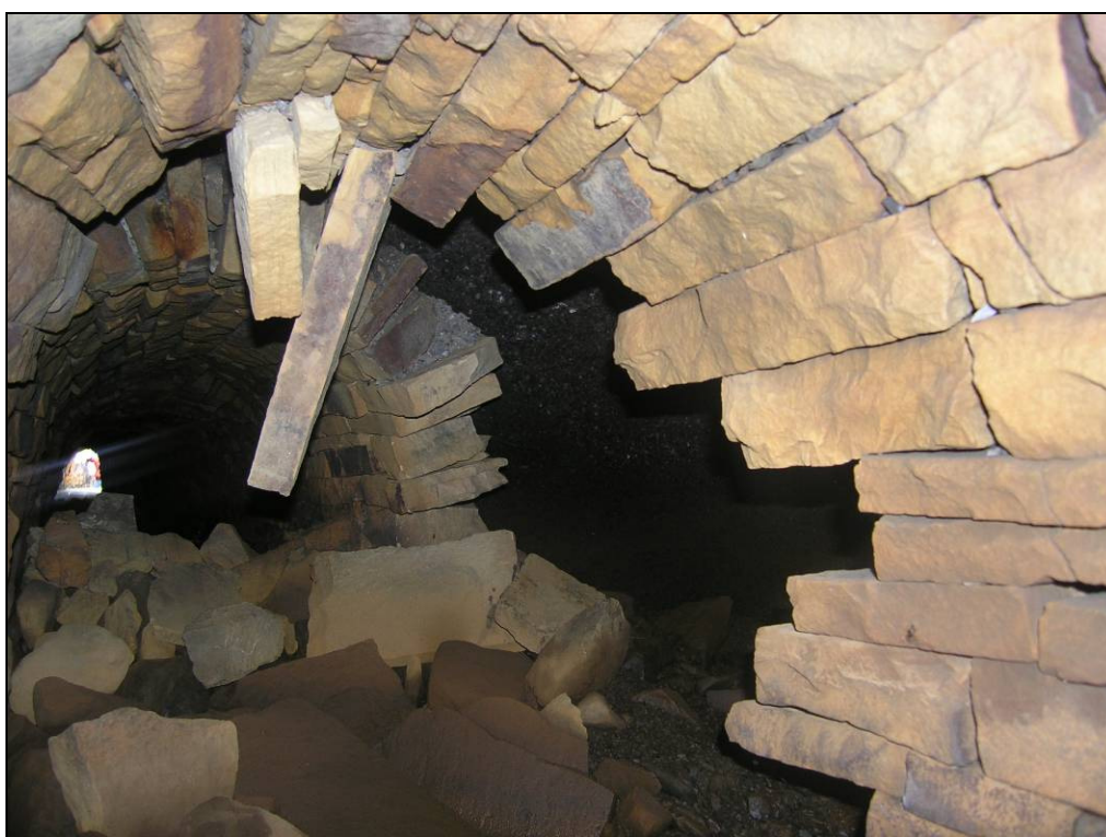
Plate 12: Collapsed section of culvert (2462). Note large void behind collapse.
