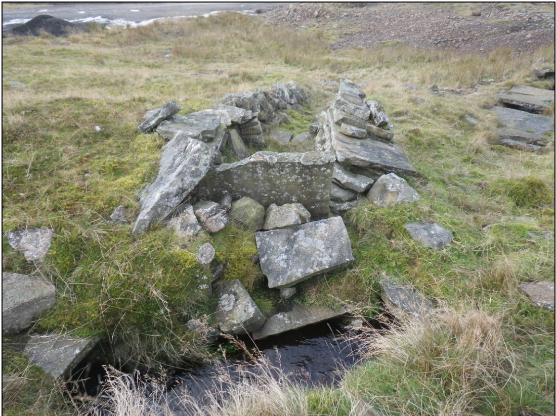
Plate 20: Overflow (2617) with the continuation of leat (0010) to the right of the image.
