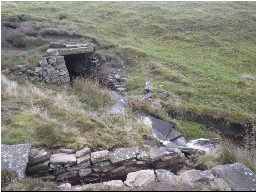
Plate 56: Water from sluice (2578) flowing through the junction between culvert (2440) and culvert (2439).
