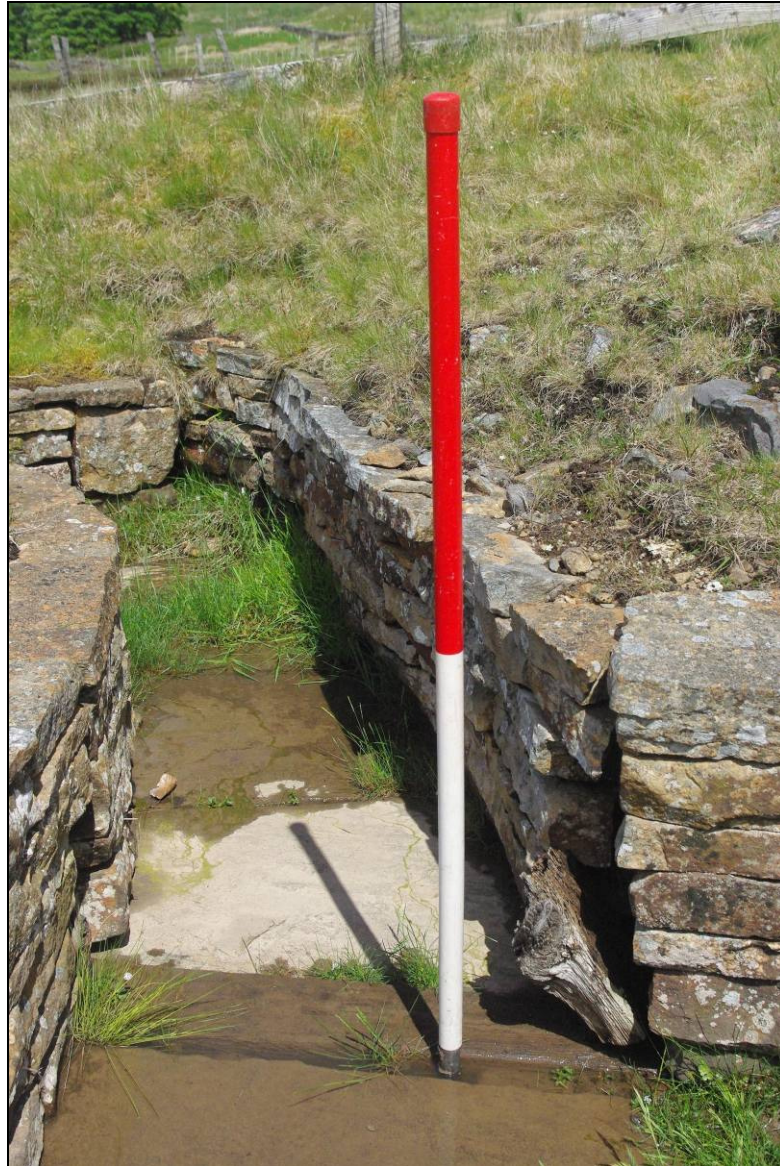
Plate 44: Sluice gate (2629) with the start of leat (2572) at the top of the image.
