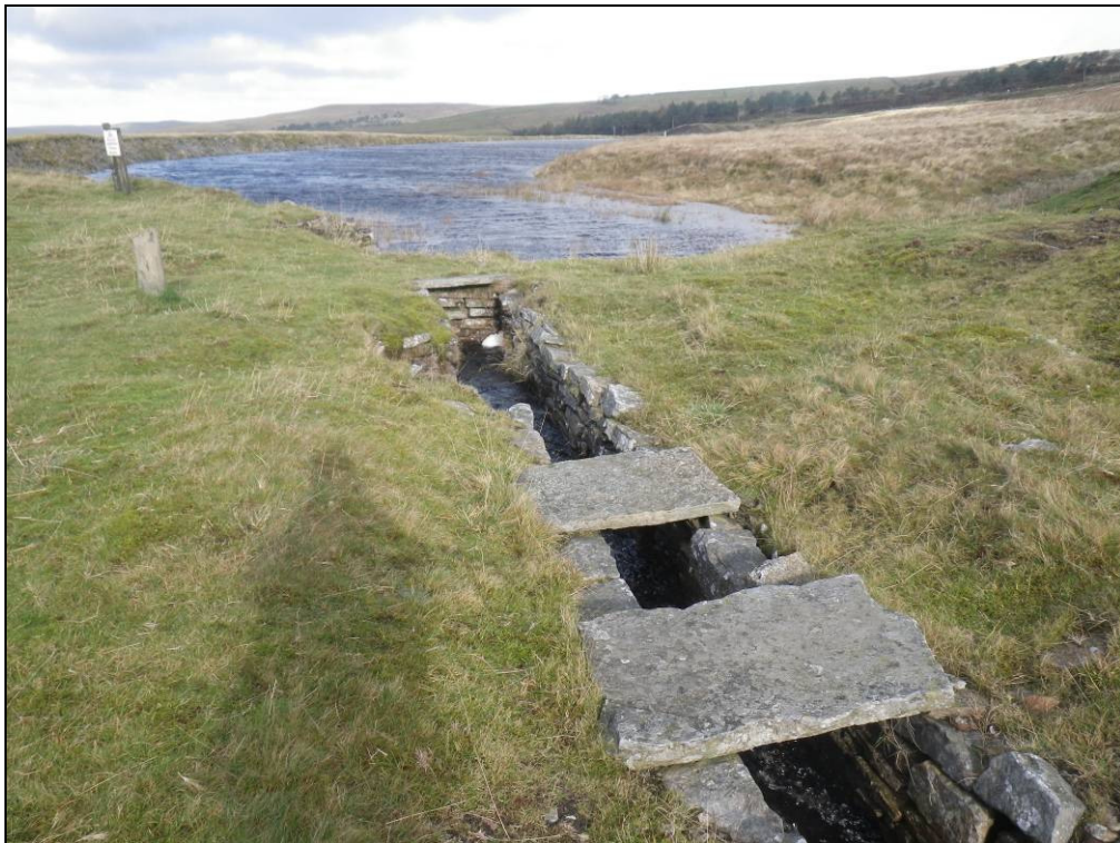
Plate 19: Leat (0010) feeding into the south end of Handsome Mea. Overflow (2580) at the top end of the leat.
