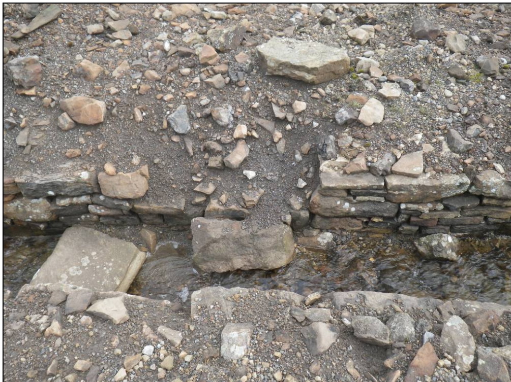
Plate 32: Collapsed section of side wall.
