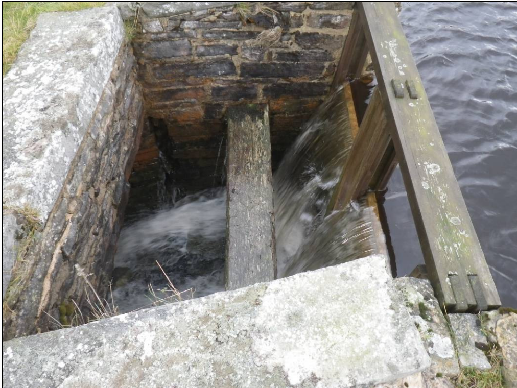
Plate 55: Sluice gate (2578) after a heavy period of rain. Note wooden sluice is in the down position.
