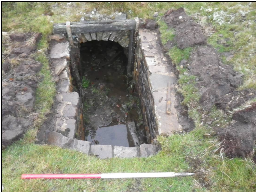
Plate 41: Sluice gate (2628) with pipe (2525) entering the sluice to the left of the image.
