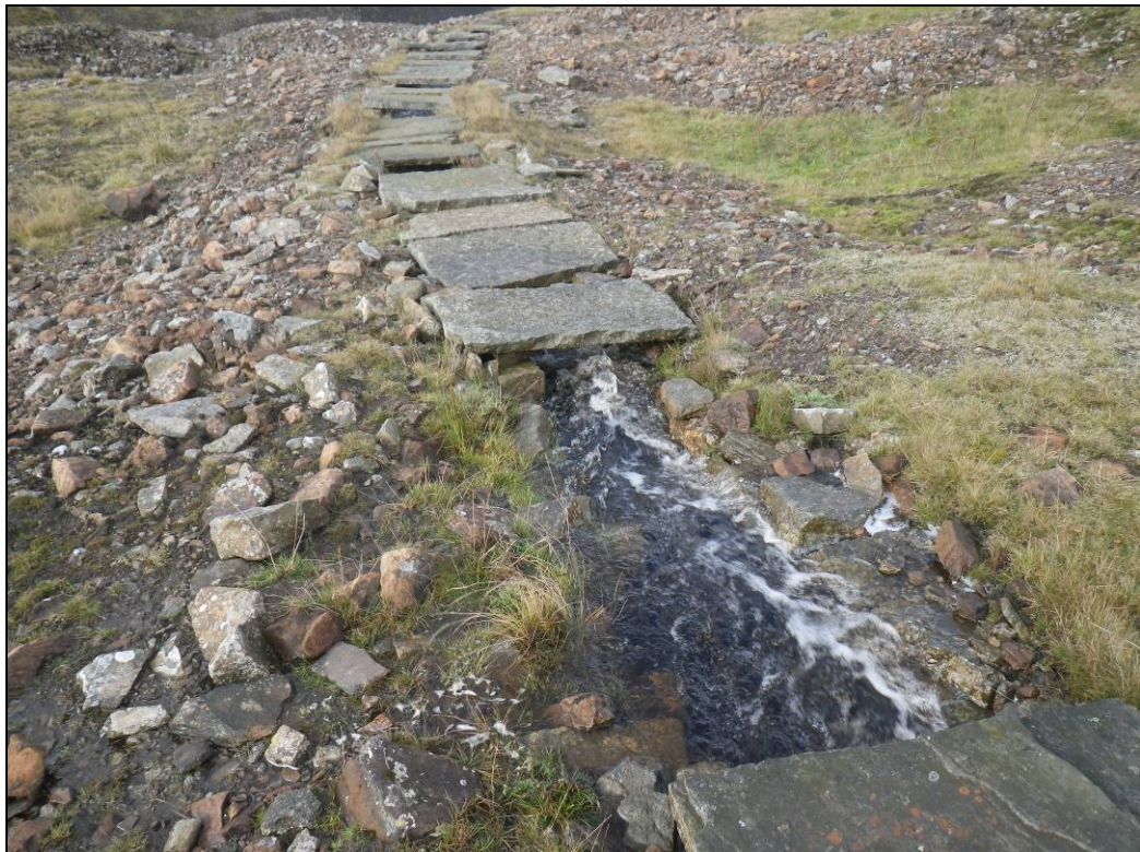
Plate 23: Leat (0010) struggling to cope with amount of water flowing through it. Notice water flowing out of the leat to the left of the image.
