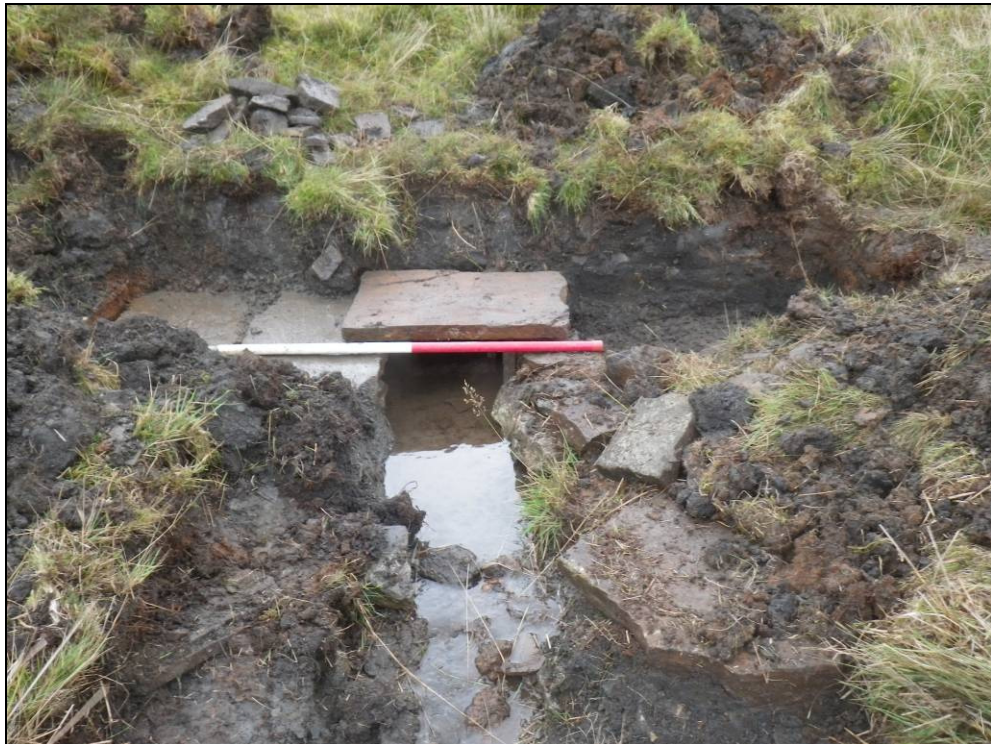
Plate 13: Trench 1 showing leat (0029) diversion facing northeast.
