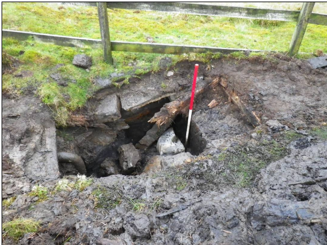
Plate 47: Mid-excavation shot of collapsed support beam.
