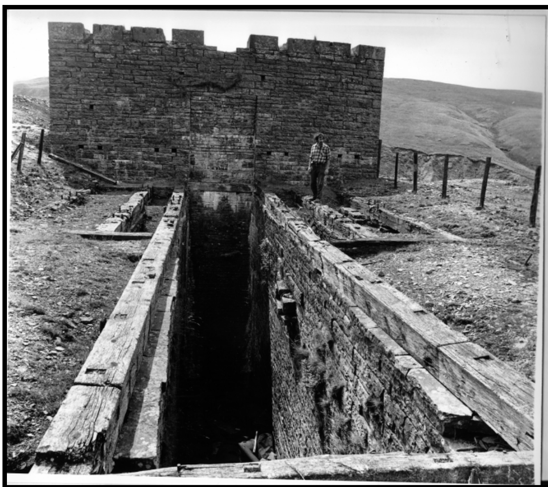
Fig 4. The Stagg Condenser wheel-pit in 1975 (© NMCS archive).
