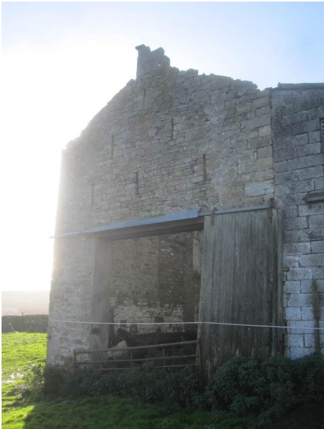
Phase Four changes to traditional range. New openings in east gable of former byre and hayloft (left) and bastle south wall ((right)
