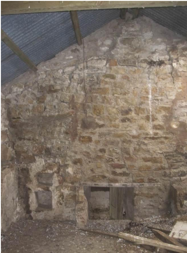
Bastle: first floor west gable showing top of fireplace, salt boxes and inserted doorway (left) Bastle: exterior of west gable with fine squared coursed rubble with offsets, vent and inserted doorway (right)
