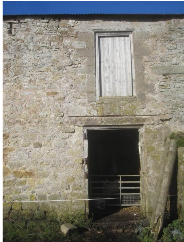
Phase Four changes to traditional range. New openings in east gable of former byre and hayloft (left) and bastle south wall ((right)
