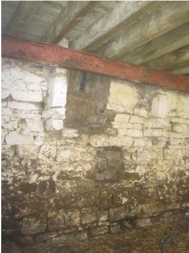
Ground floor of bastle; west wall showing byre vent, first floor fireplace and later opening cut through to store (left). North wall of bastle at east end showing later house built over gable end and later raising of bastle to same height (right)
