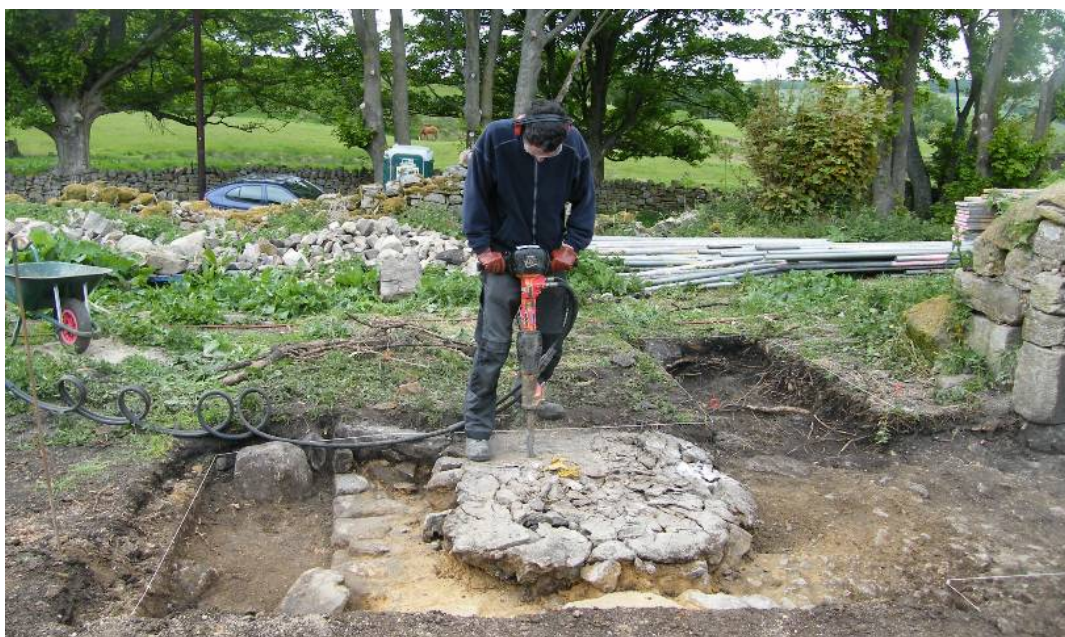
Plate 5.2 breaking the concrete pier base 1004, looking north
