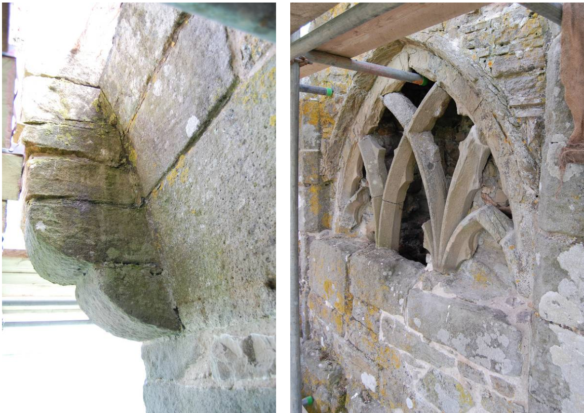
Plate 4.8 The SE angle tower of the chapel, upper parts showing arch springing on its north side
