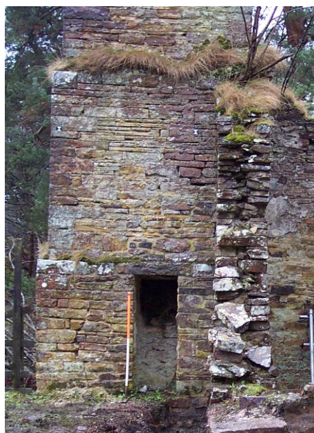
Plate 8 Example of similar stoke-hole opening in chimney of upstanding Engine House to the W
