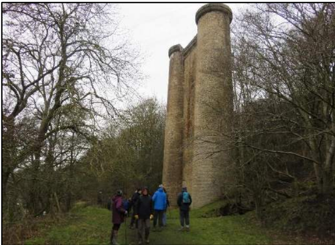
Fig.2: Lands viaduct crossing the River Gaunless designed by Sir Thomas Bouch and opened in 1863
