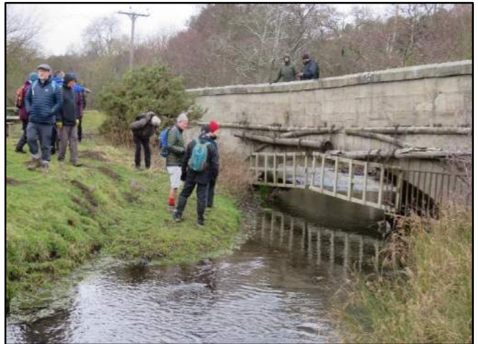
Fig.3: Skew Bridge built without a keystone
