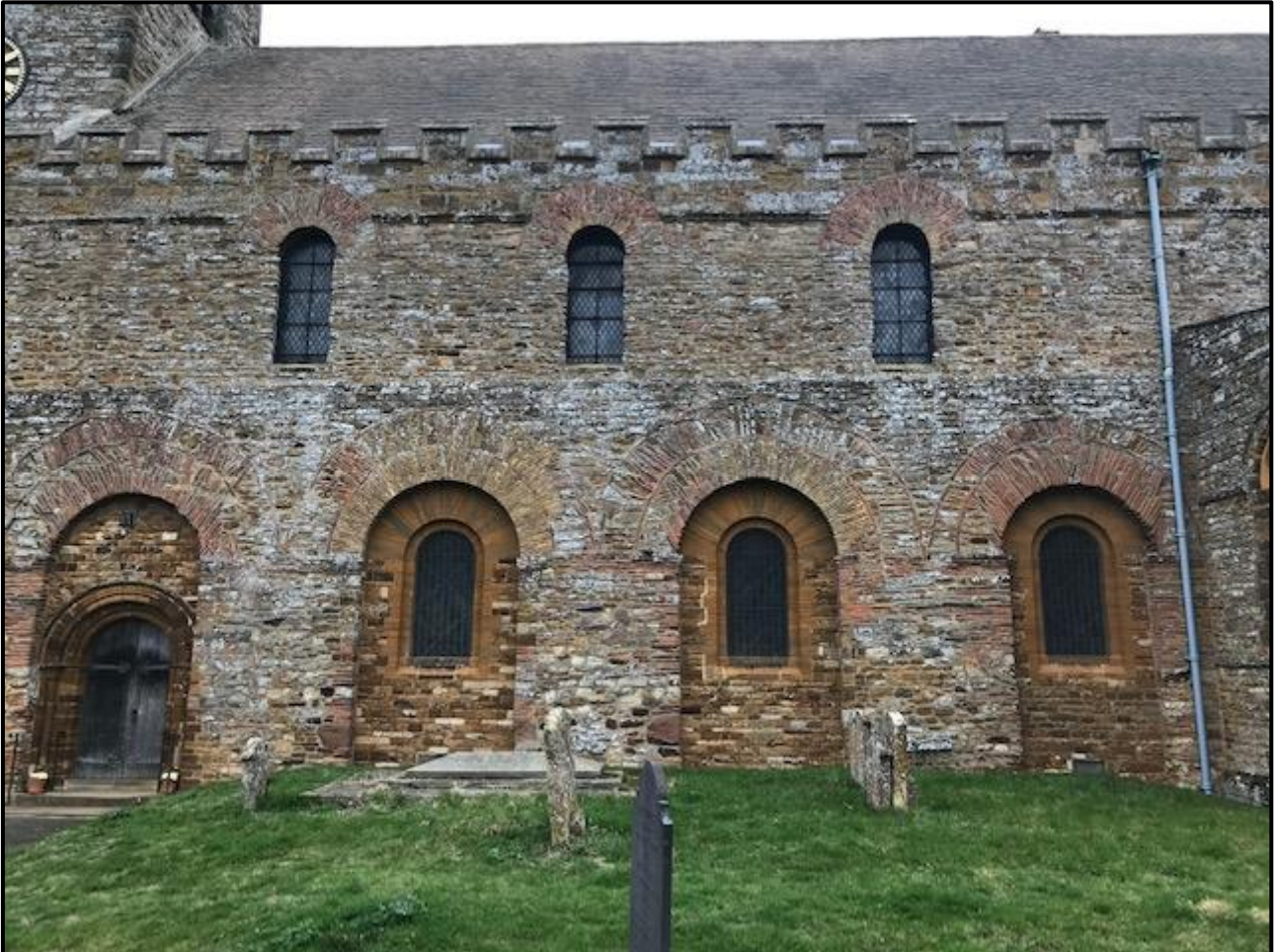
Fig.2: A large section of the nave south wall
