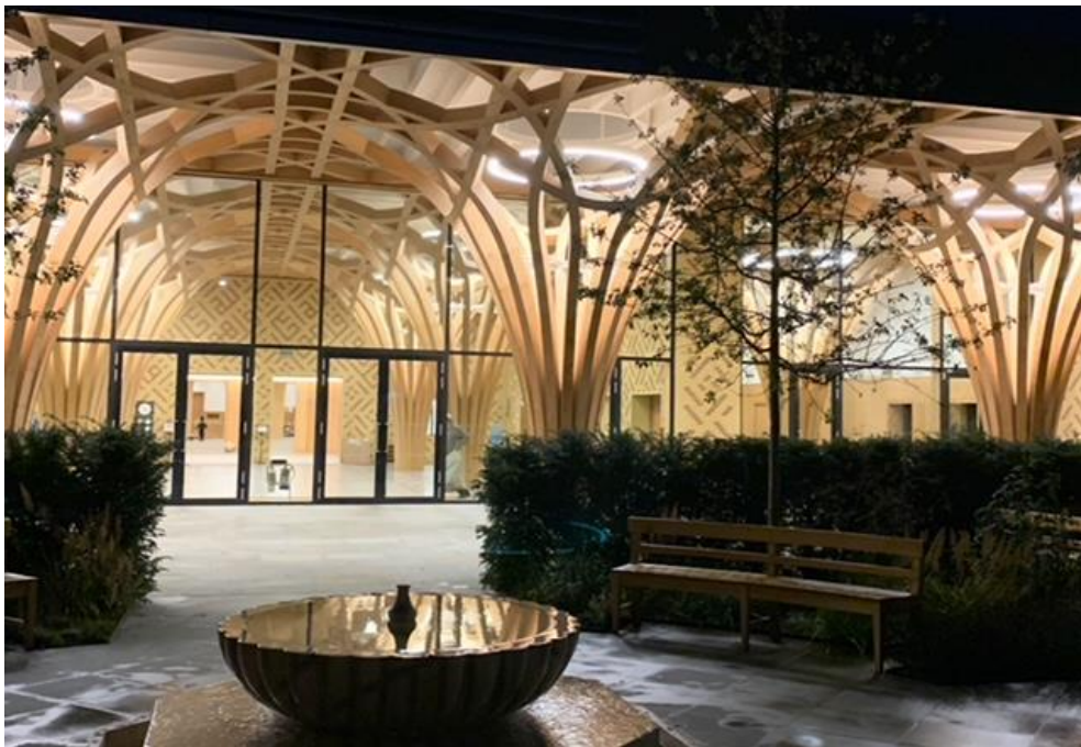
Fig.3: Cambridge Central Square showing the remarkable timber tree-like columns
