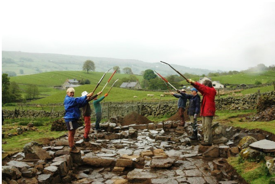
Figure 59: Members of AA standing on the padstones to demonstrate the crucks of building F9.
