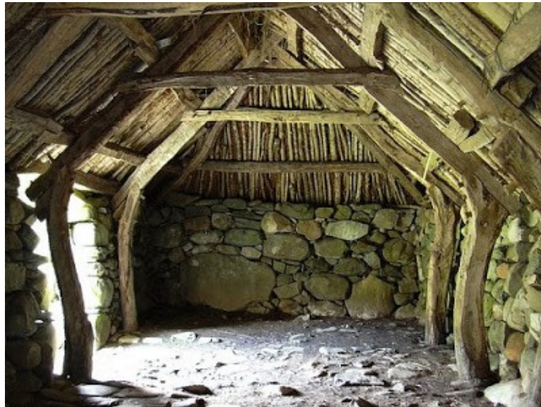
Figure 61: Building at Auchindrain (Scotland) with a cruck frame and hipped roof. Note padstones. Preserved at the Auchindrain Township Museum: http://www.auchindrain.org.uk .
